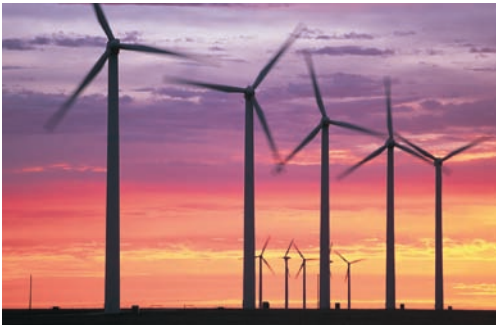
Wind turbines typically have two or three long blades that spin when the wind blows. The spinning movement is then used to turn a generator to produce electricity.
