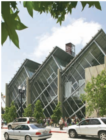
Photovoltaic panels on slanted roof segments are barely visible on The New Children's Museum. The central glass chimney seen on top serves as a cooling tower, exhausting hot air from gallery spaces.
