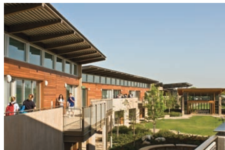
At Francis Parker School, a narrow footprint, deep overhangs, sunshades, light shelves, and louvers redirect light deep into the classrooms through spectrally selective glazing with high visible light transmittance.
