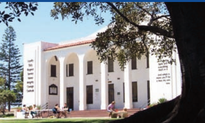
The Army and Navy Academy installed energy-saving lighting with help from SDG&E's On-Bill Financing program.
