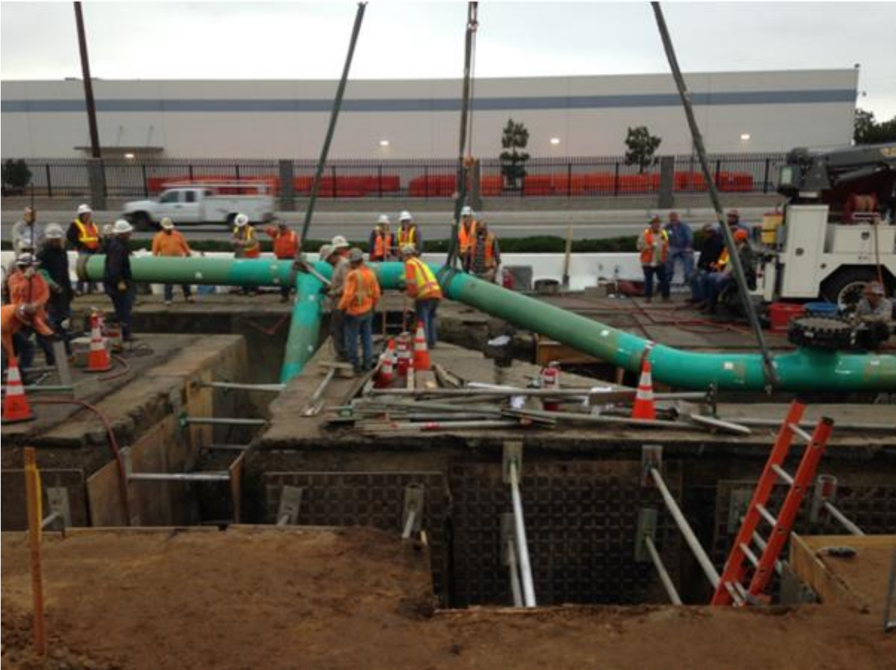
Figure 9: Lowering Section of Pipe into Trench
