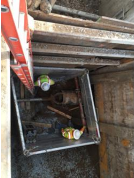
Figure 7: Jack and Bore Pit
