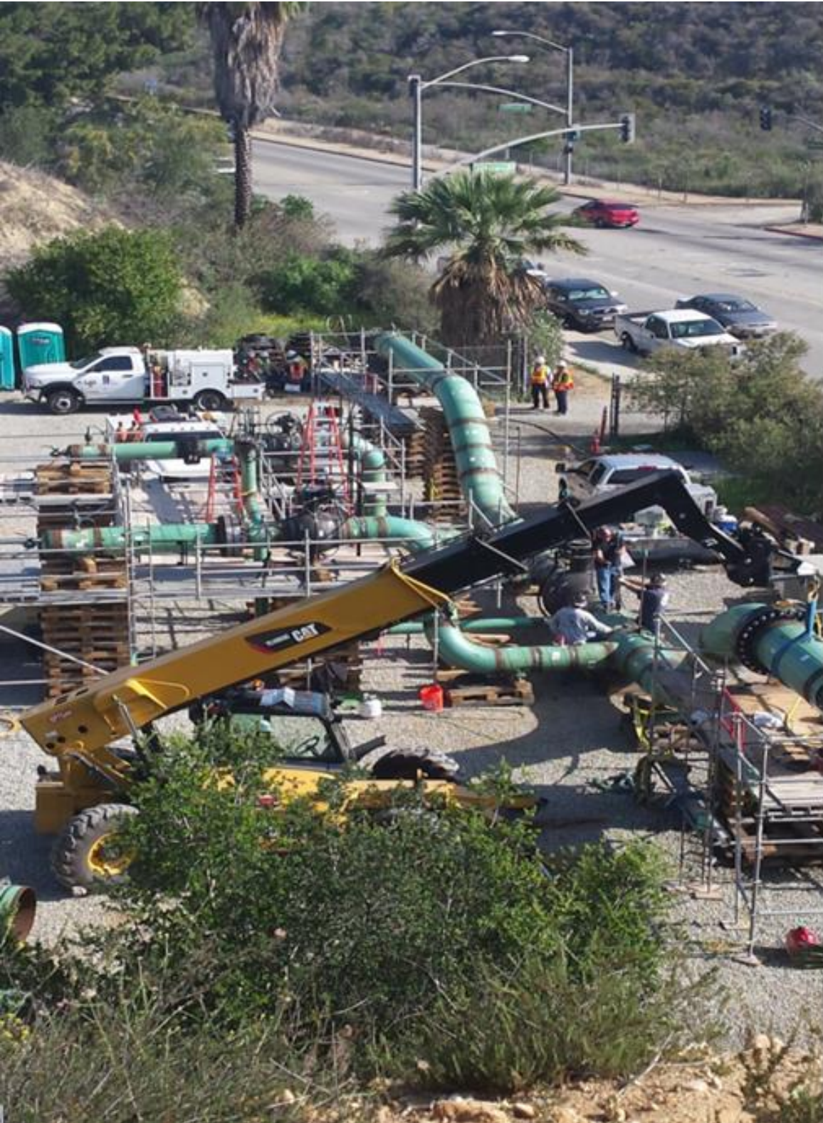
Figure 10: Above-Ground Pre-Fabrication of Valve Assembly
