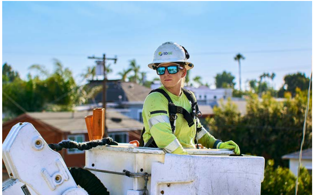
The existing wood structures will be replaced with new fire-resistant steel structures.
