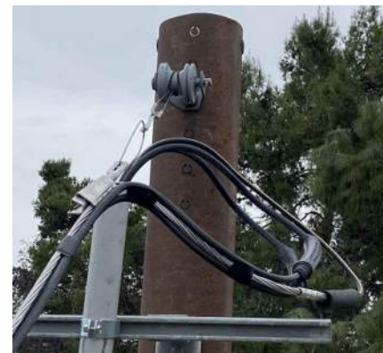
FIGURE 4 STORM SAFE FLEXIBLE BAIL ASSEMBLY
