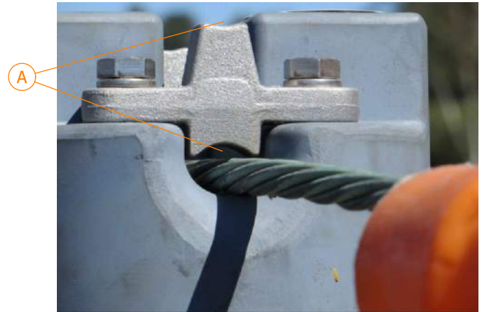
FIGURE 2 INCORRECT INSTALLATION
