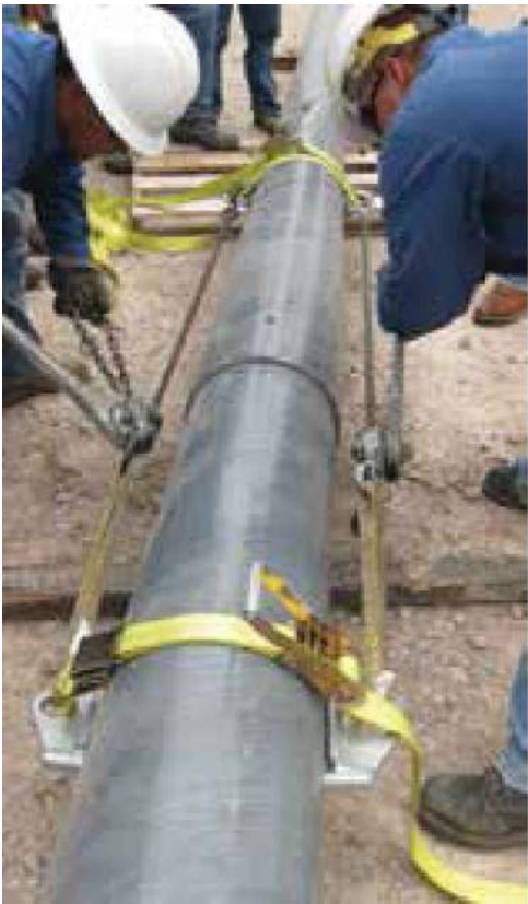
FIGURE 12 COME-ALONG INSTALLATION
