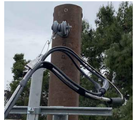
FIGURE 4 STORM SAFE FLEXIBLE BAIL ASSEMBLY
