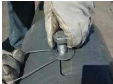
FIGURE 15 BOLT AND WASHER INSTALLATION
