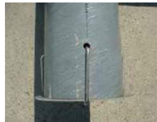
J-BOLTS ON OUTSIDE OF MODULE
