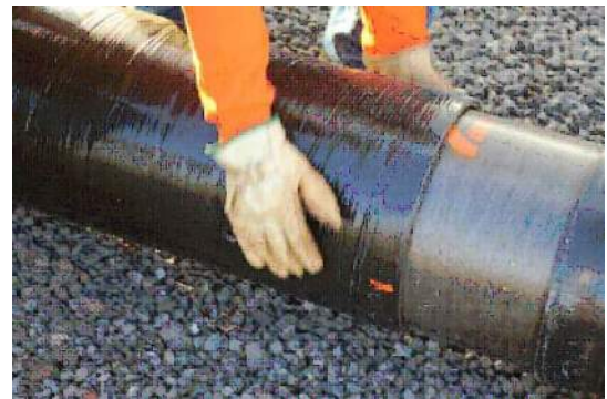
FIGURE 8 ALIGNING SECTIONS (J)
