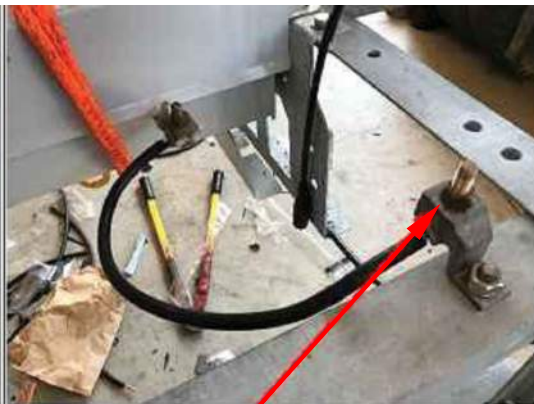
GROUND SWITCH FOR SWITCH FRAME
