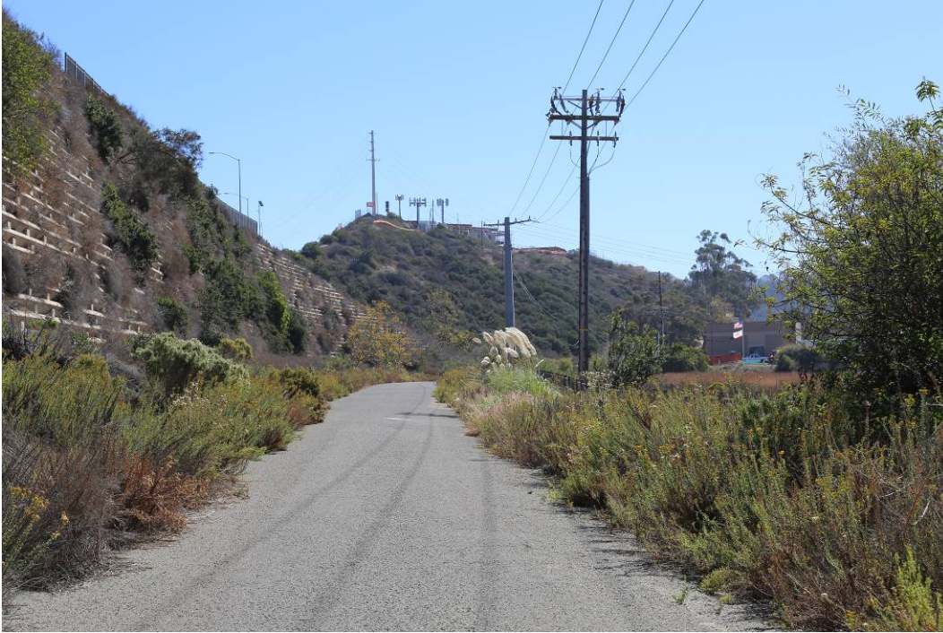
Photograph 9: Existing view looking south-southeast along the Sorrento Valley Pedestrian/Multi-Use Path adjacent to Interstate 5.
