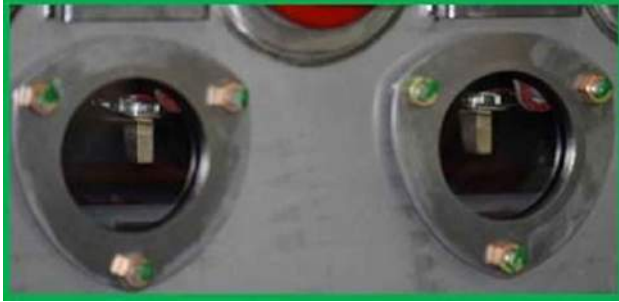
VISIBLE OPEN SHAFT "OPEN"
