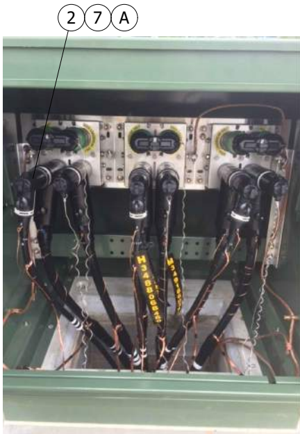
FIGURE 2 600A AND 200A COMBINATION
