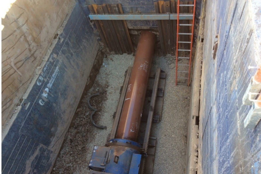
Figure 147: Boring Machine Pushing Casing Pipe
