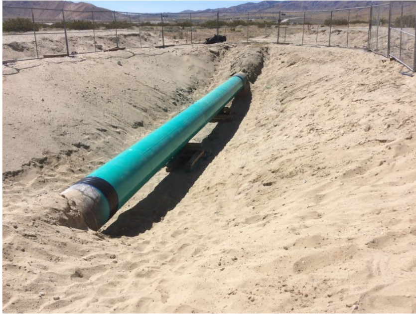
Figure 9: Pipeline Excavation and Repair Site
