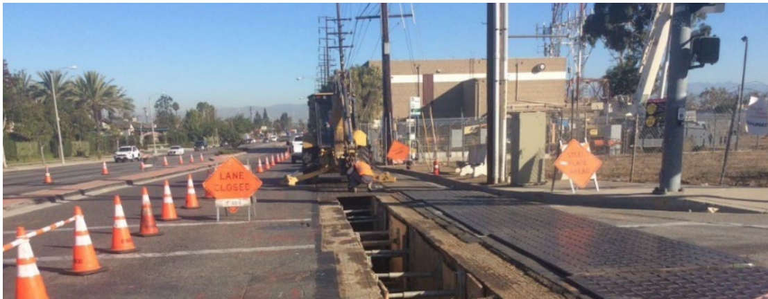
Figure 1: Traffic Control Lane Closure
