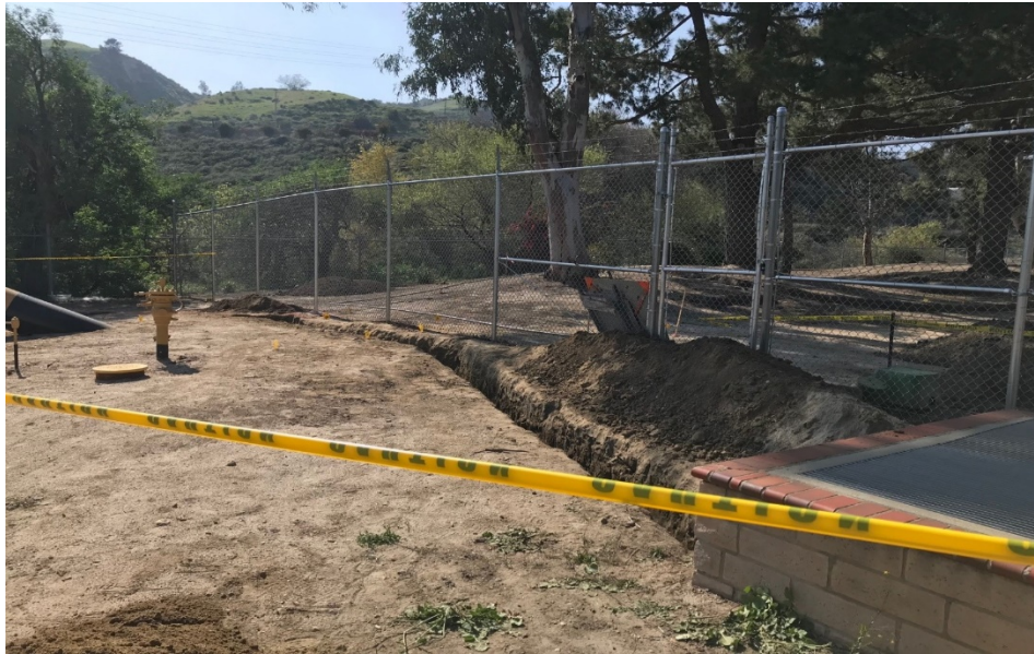
Figure 8: Hand Dug Trench
