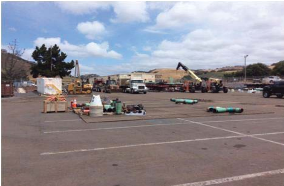
Figure 4: Construction Laydown Yard
