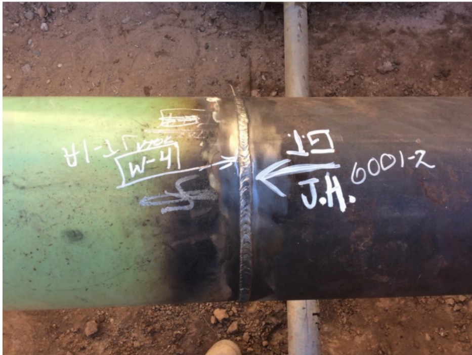
Figure 20: Pipeline Weld
