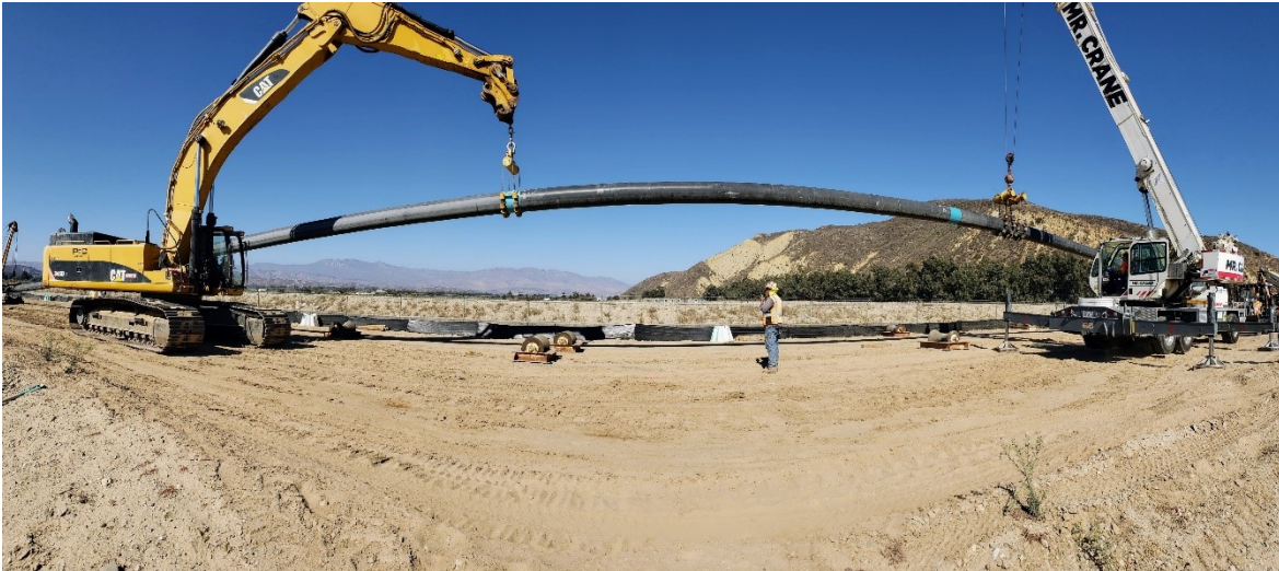
Figure 114: HDD Pullback
