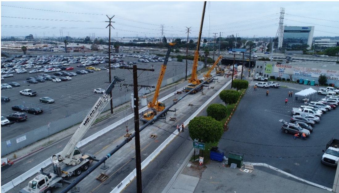
Figure 125: HDD Pullback
