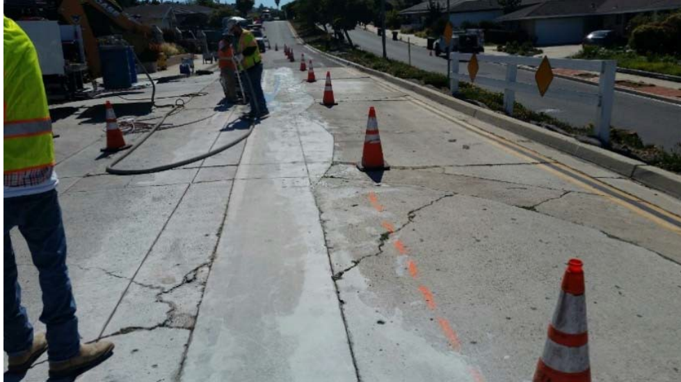
Figure 5: Saw Cutting Trench Pathway
