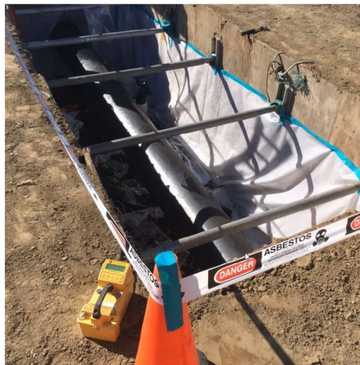
Figure 3: Typical Pipeline Abatement
