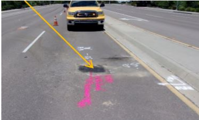
Figure 2: Potholing Location After Restoration
