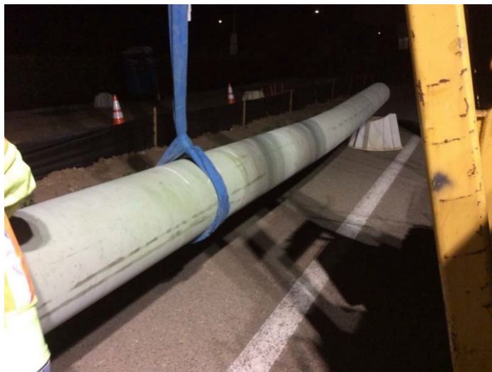
Figure 19: Pipe with Field Bend Laying on Supports
