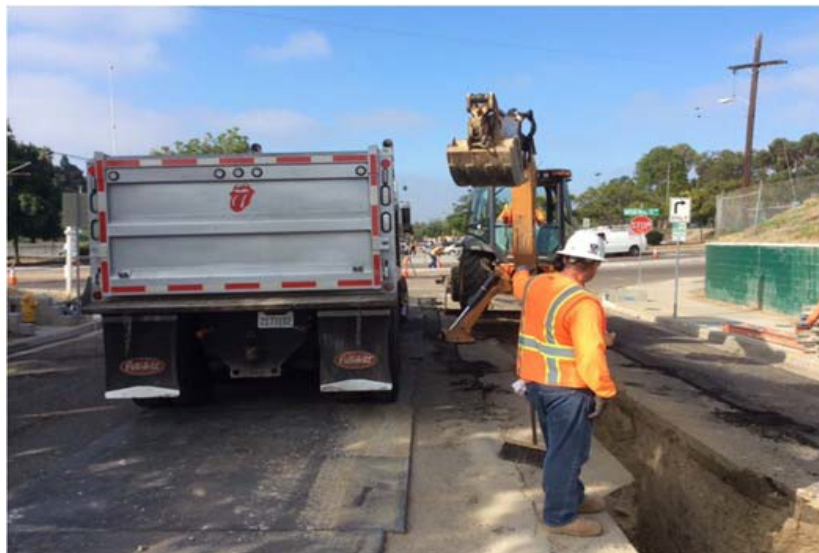
Figure 6: Trench Excavation with Backhoe
