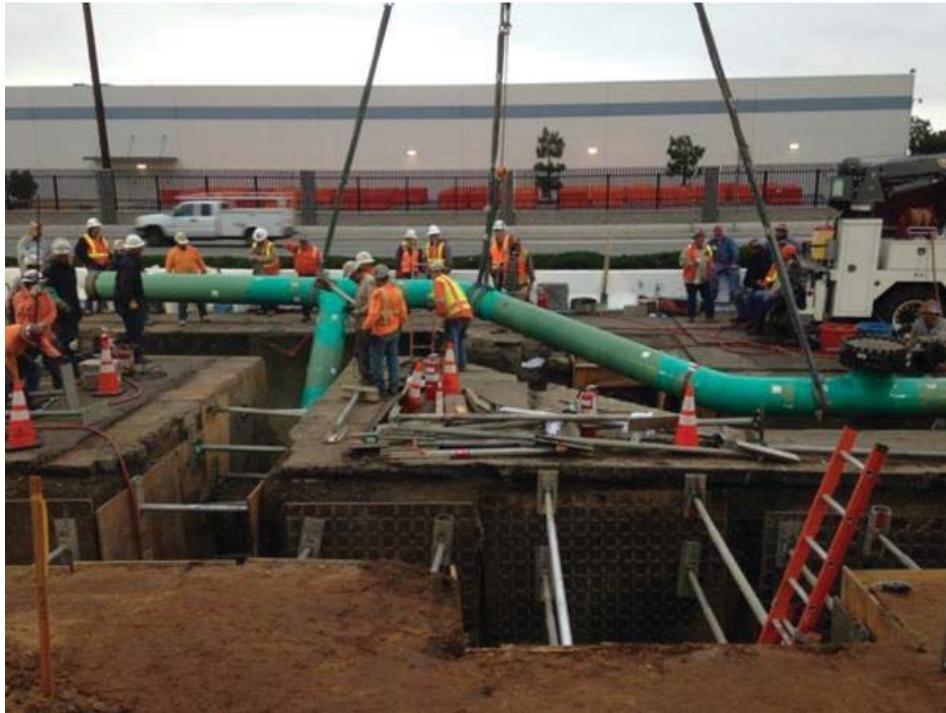
Figure 21: Lowering Section of Pipe into the Trench
